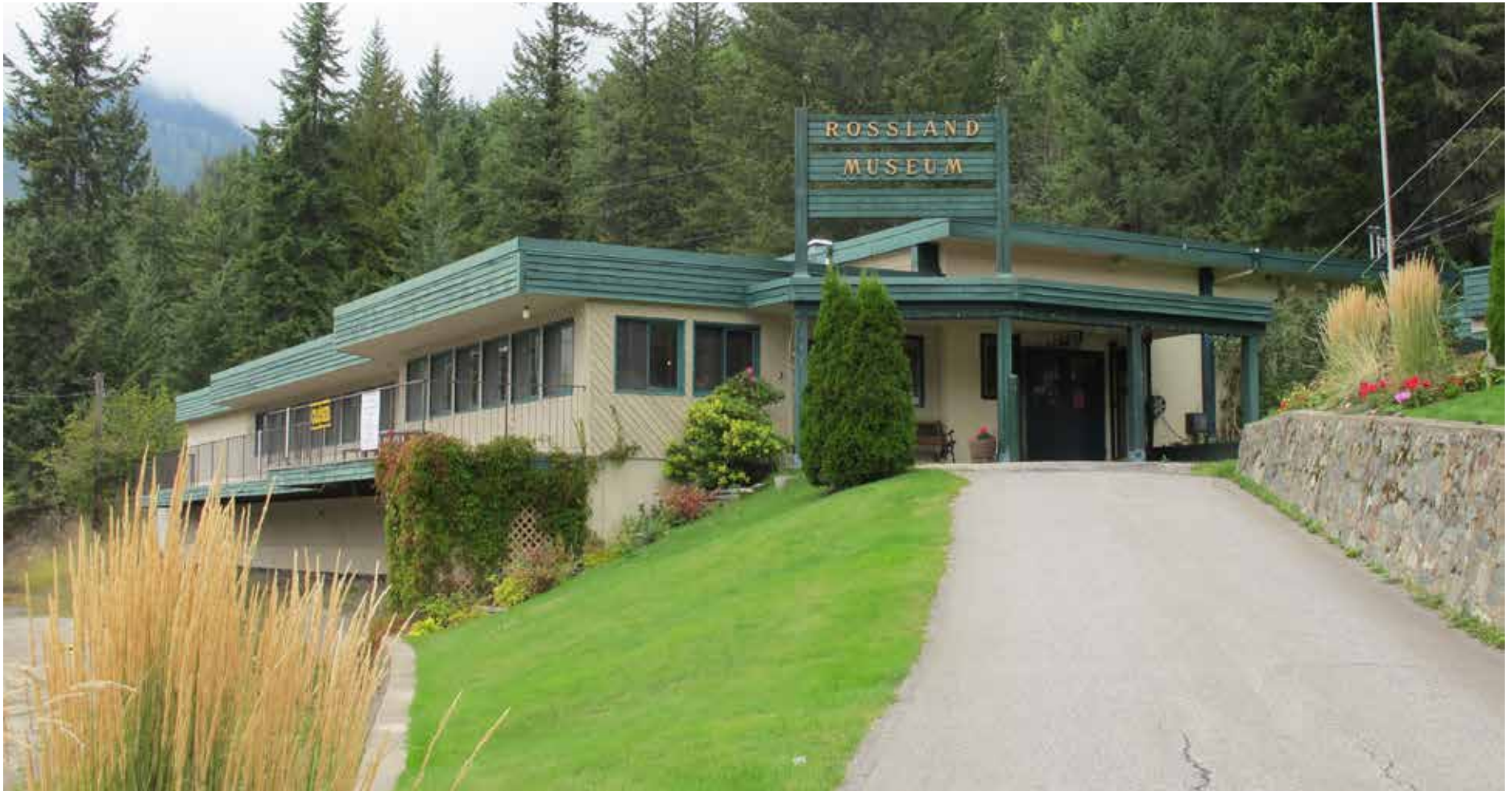
Existing entry condition.
