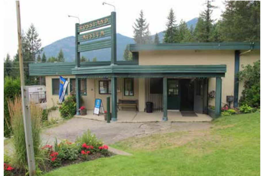
Existing condition of museum.
