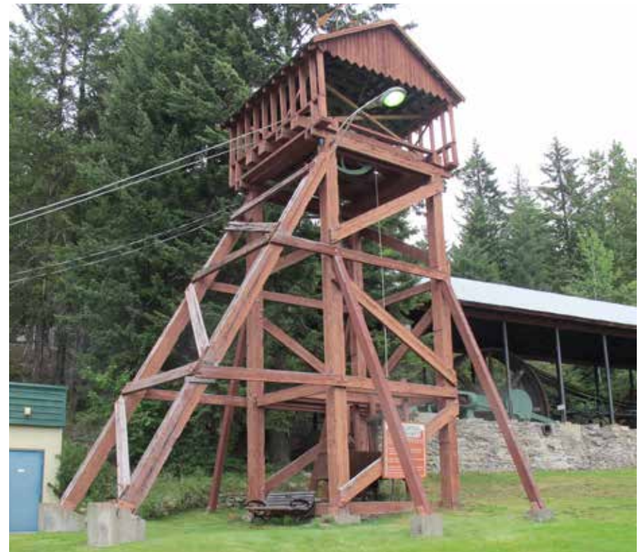
Head frame, existing location adjacent to museum.
