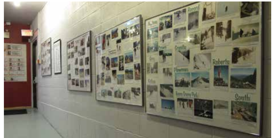
Existing concrete block wall surfaces.
